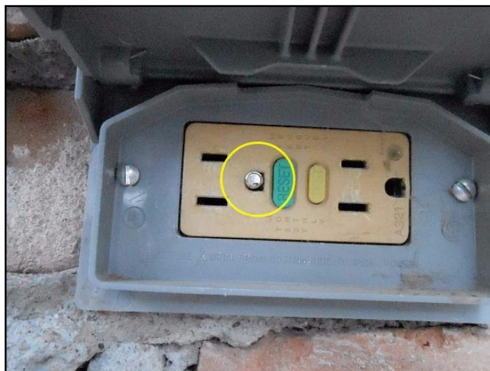
40. Broken pin or blade in slots
